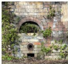
1 XBR, EXISTING BRICKWORK Repair, clean & repaint as required.
