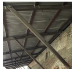
4 XTF, EXISTING TIMBER FRAMING
